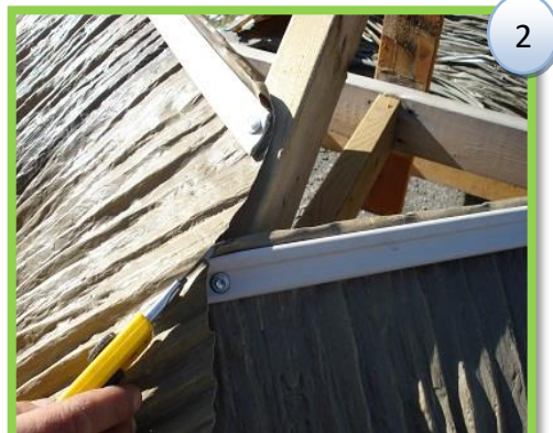
For Bora Bora/Aloha, cut the edge of the leaf at the junction from the top rail along the rafter and up to the top of the row below.
