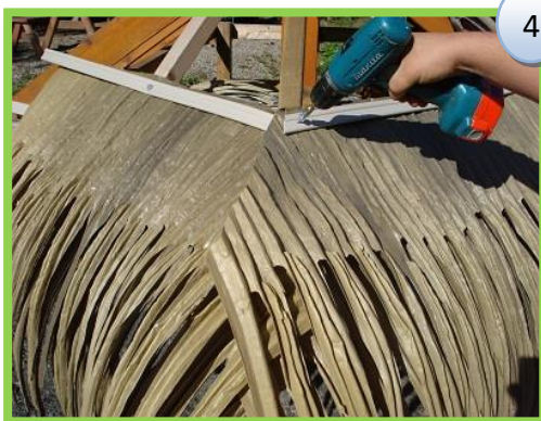
For the other side of the same junction, cut with an angle starting from the top to the end of the leaf.
