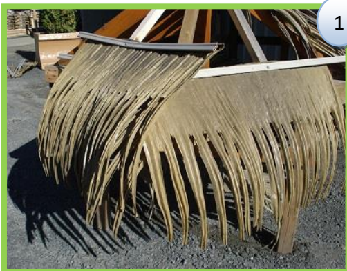
Fix the hips/valleys gradually with the leaves.
