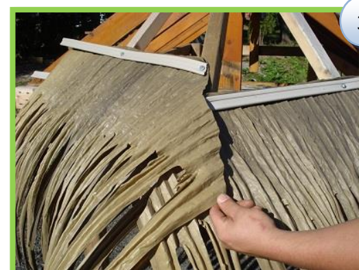
From that point, cut the leaf with a slight angle to cover the leaf from the opposite side of the row below.
